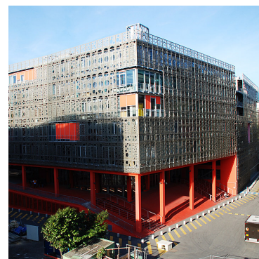
The Atrium facade opposite to the metro
